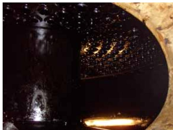
Oily matter get into boiler from damaged heating coils of fuel oil heaters, lubricating oil heaters, fuel oil tanks or waste oil tanks. When oily matter is detected in boiler, it is important to specify the place where oil leaks, and repair it.
