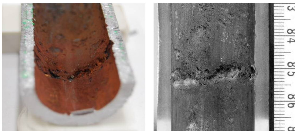
Corrosion of feed water nozzle caused by sulfate ion
