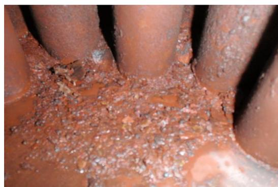
Accumulated sludge on boiler bottom side
